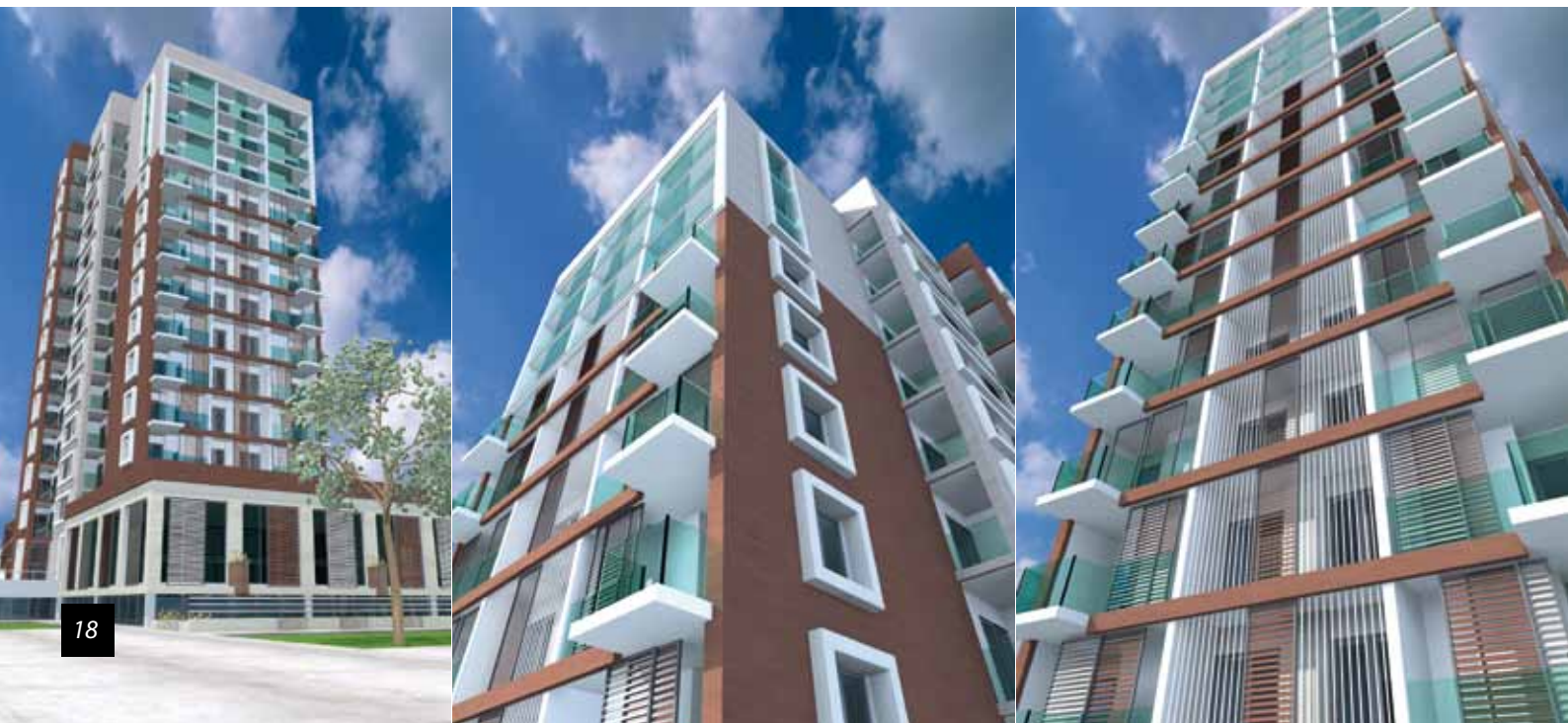
Hotel "LIGHTHOUSE of Montenegro" | ul. Norveška br.2 Igalo, Herceg Novi ( bivši Hotel "Metalurg") | Investitor : "LIGHTHOUSE of Montenegro" doo Herceg Novi
